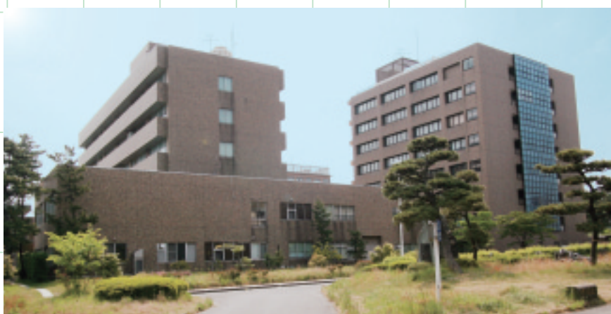
共通管理棟（左）と情報理工棟（右）。 [Main Building (left) and Information Science and Engineering Building (right)]
